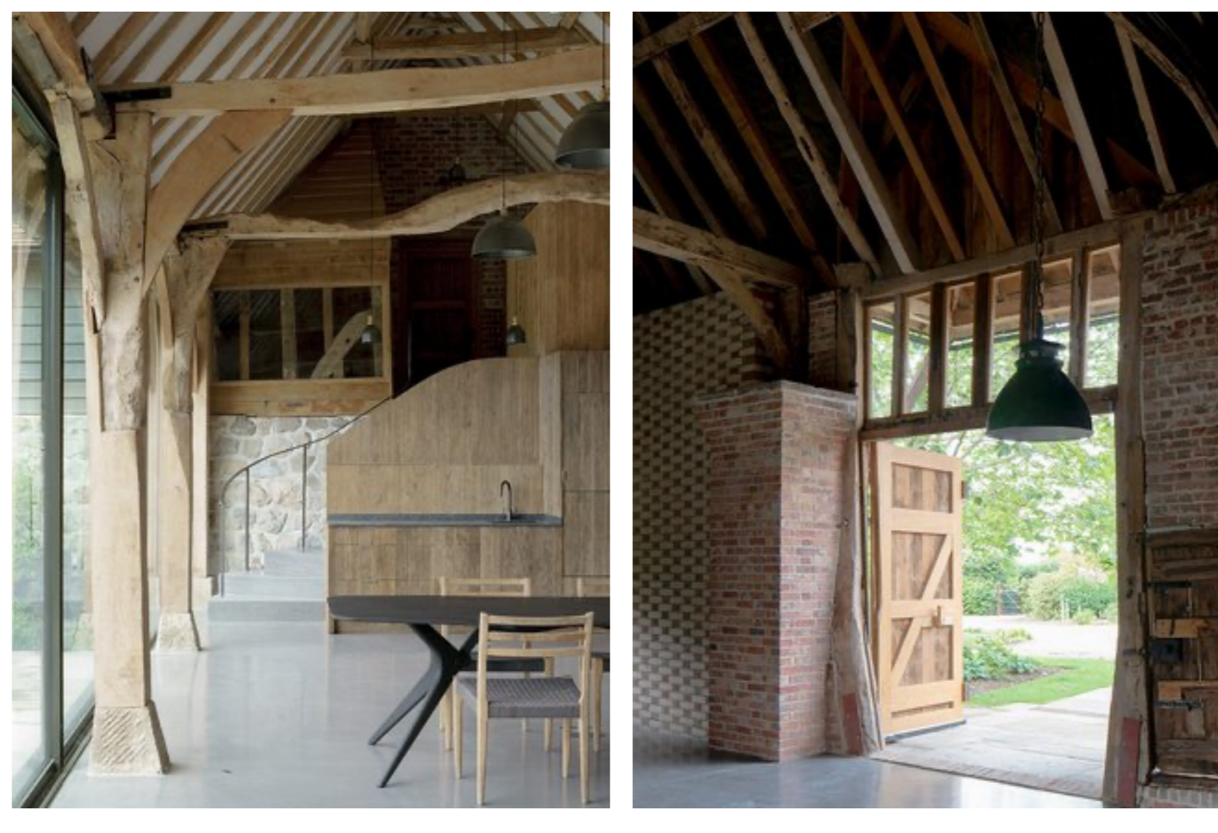
Original brickwork and a ragstone wall are exposed in the long barn. Credit: Building Narratives
